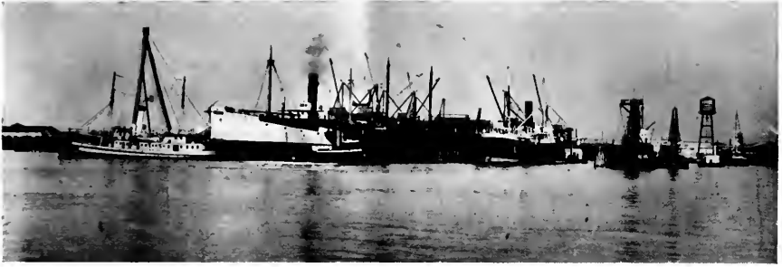
Waterfront of the Moore and Scott Iron Works' plant, Oakland, California.
